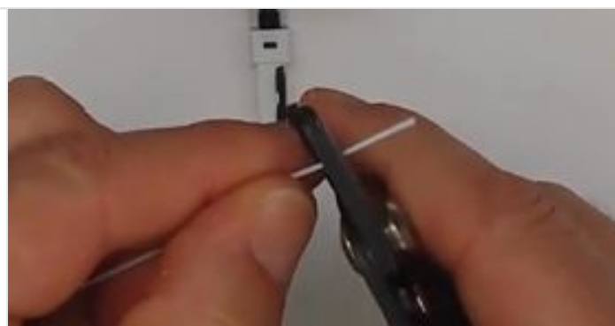
Strip approx. 50mm. Primary coating must be removed
